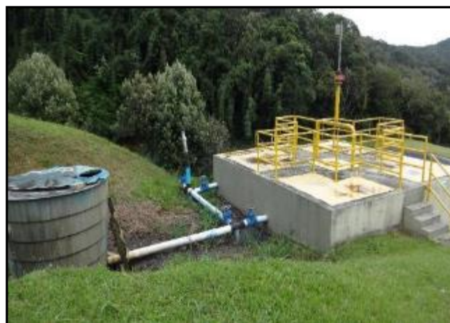
Figura 19: Reator UASB.
